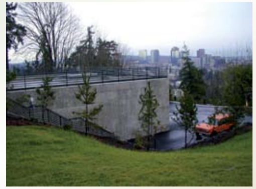
The new Meydenbauer Reservoir was designed to blend into a hillside for minimal impact to the neighborhood.
