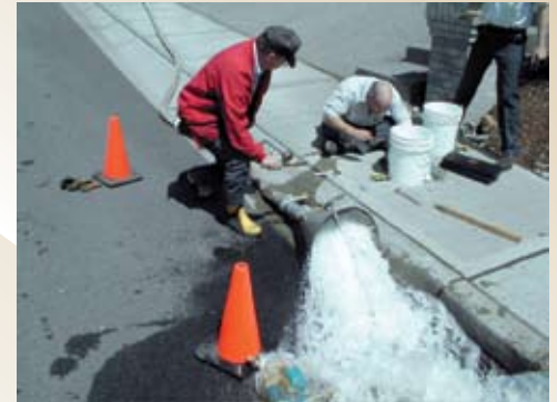
To improve water quality, Bellevue flushes about 20 percent of its system each year.
