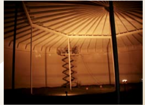
Improvements were made inside the three-million-gallon Factoria Reservoir.
